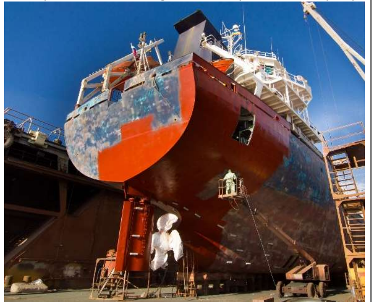
Hull repairs, Water blasting of vessel dry docked on slipway
