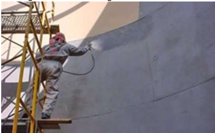
Painting of Petroleum storage tank
