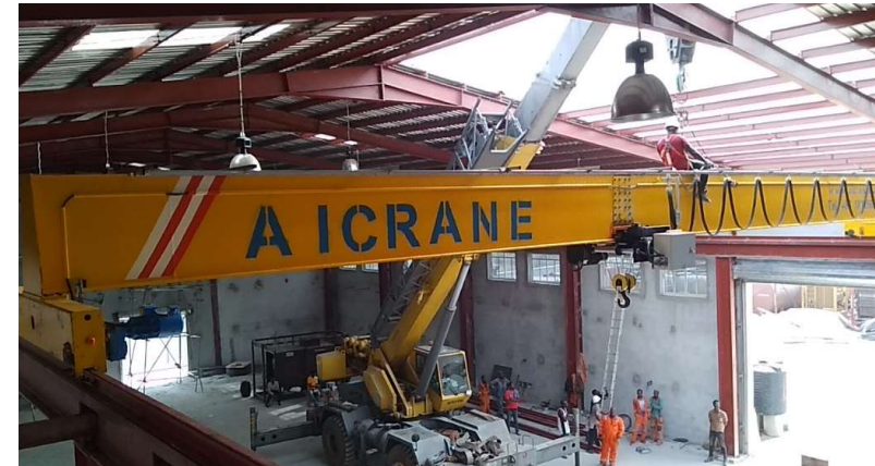
10 Ton Crane Installation on runway beams @ Topline workshop
