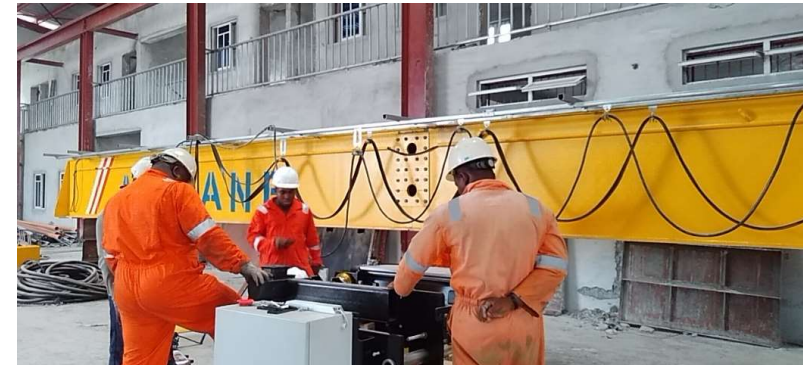
10 Ton Crane Installation on runway beams @ Topline workshop
