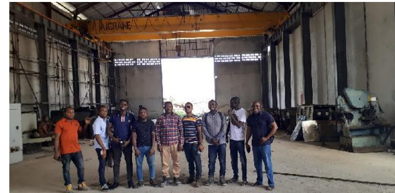
10 Ton OH Crane: Mechanical assembly of parts and wiring on ground
