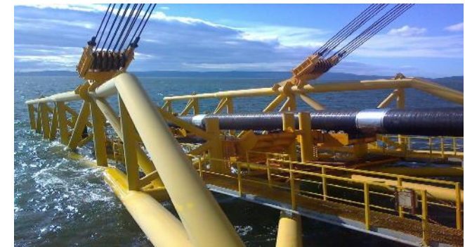
Installation of Pipeline mattress
