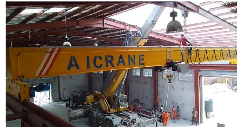
10 Ton Crane Installation on runway beams @ Topline workshop
